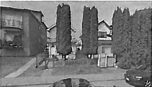
Existing along Albert
