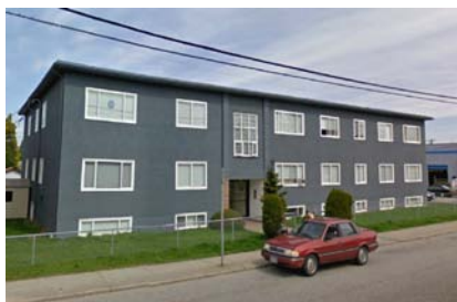
Existing Low Rise Apartment
