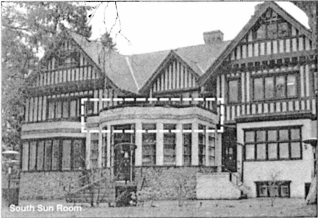
Hart House Areas of wall and stucco restoration
