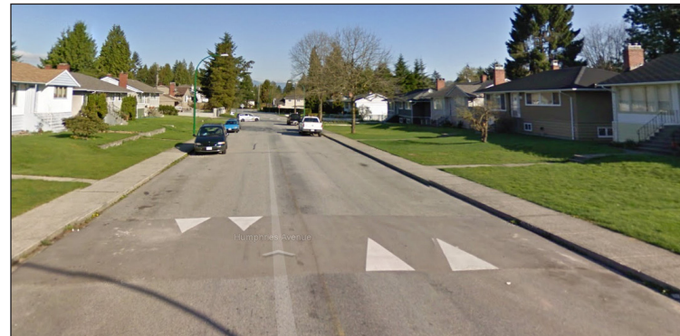
A speed hump on a residential street
