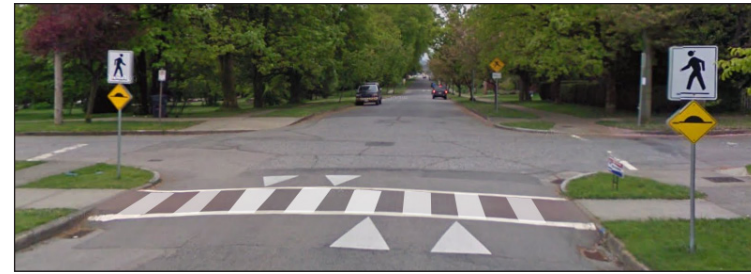
A raised crosswalk
