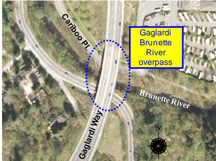
Figure 1: Gaglardi Way Brunette River Overpass
