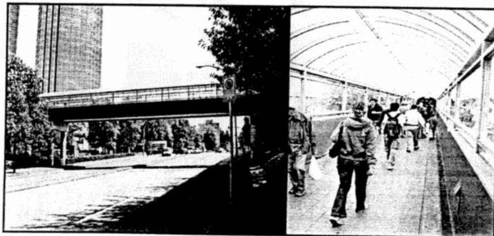
Figure 6 Existing Metrotown Passarelle
