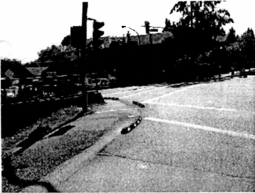
North-East Corner Of Douglas Road & Sprott Street With Temporary Rubber Barrier Curbs.
