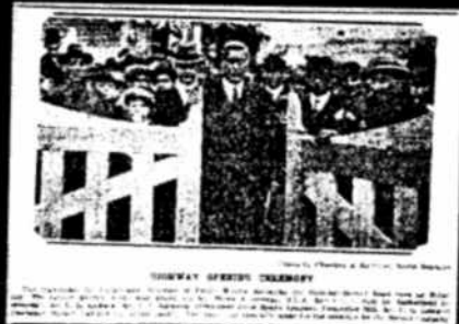
The paving of Hastings-Barnet Highway was front page news in 1927.
