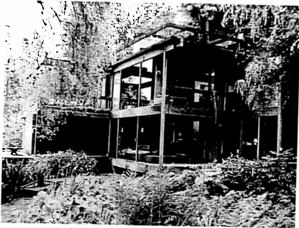
View of northwest elevation from Deer Lake
