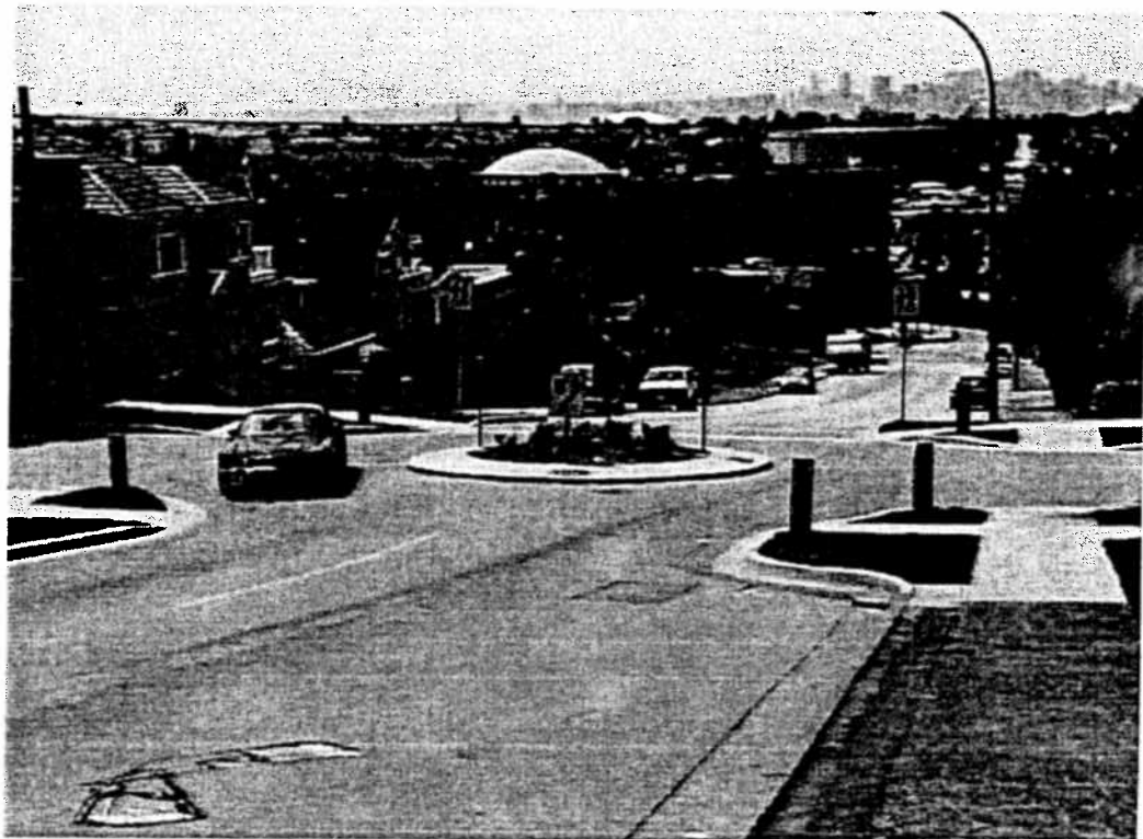
Figure 8 Traffic Circle at Skeena/Kootenay (City of Vancouver)
