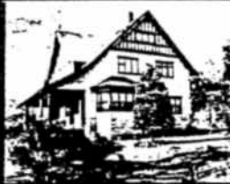
The Anderson House - side view
