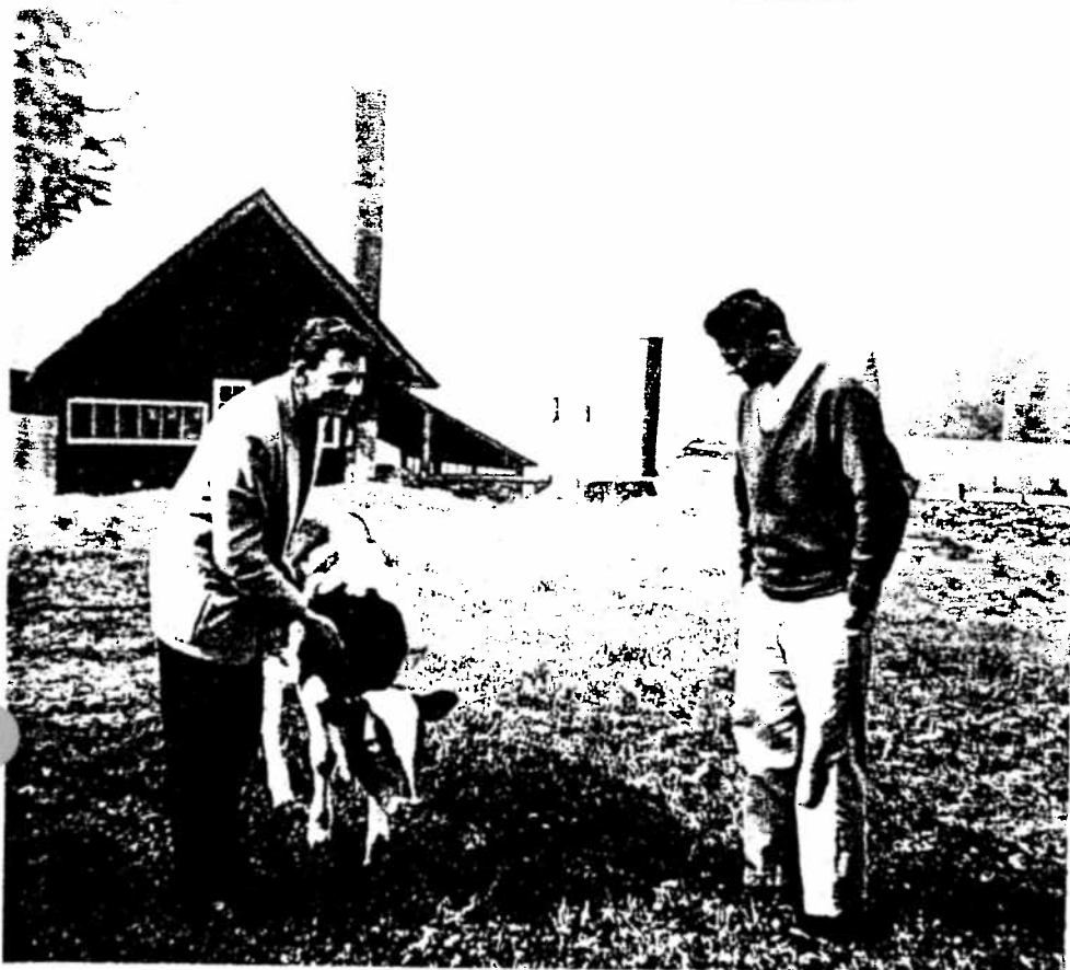
ORIGINAL STEAM PLANT: 1950'S PHOTO VIEW FROM NORTH
