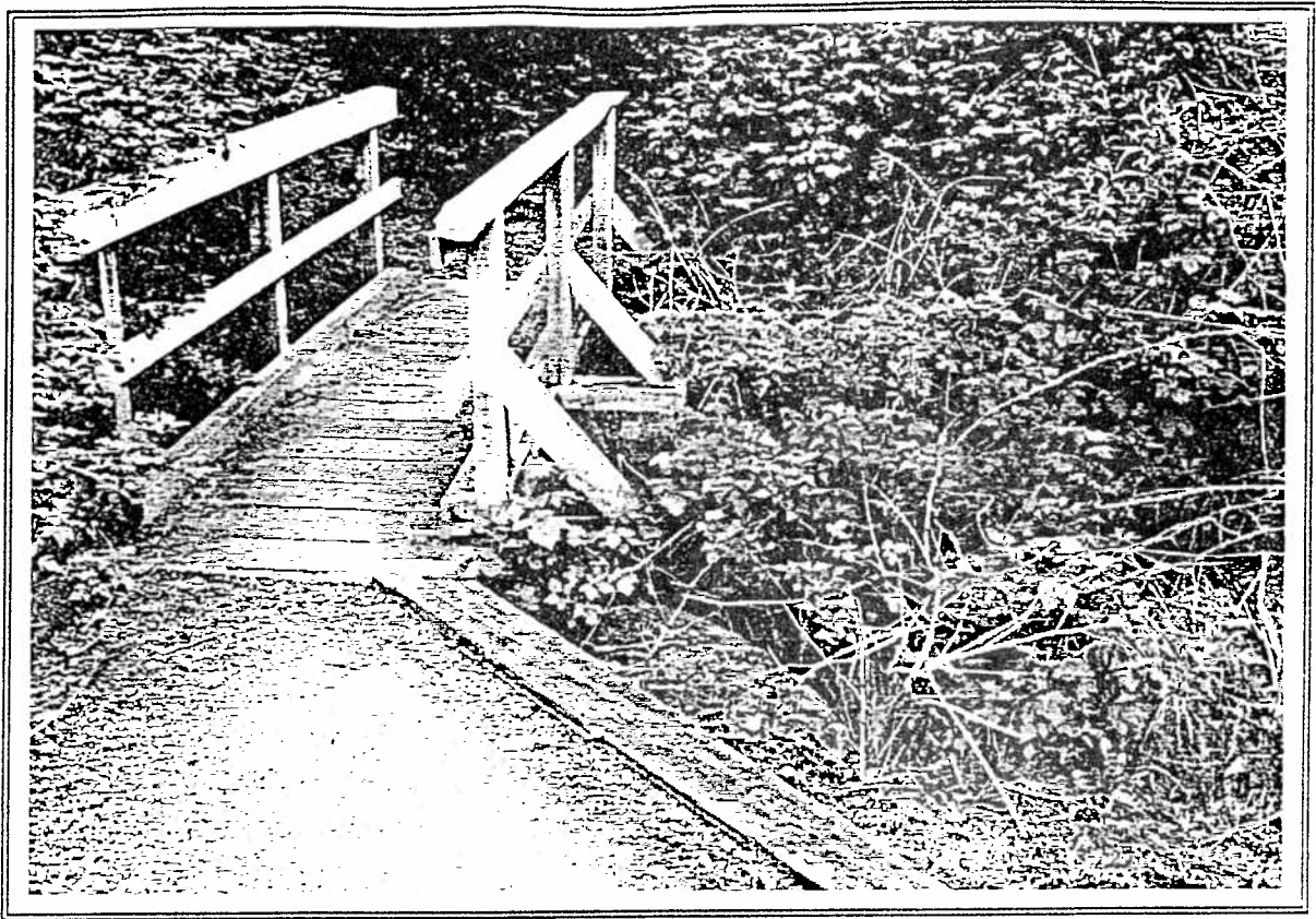
Site R3. Removal of accumulated sand below pedestrian bridge.
