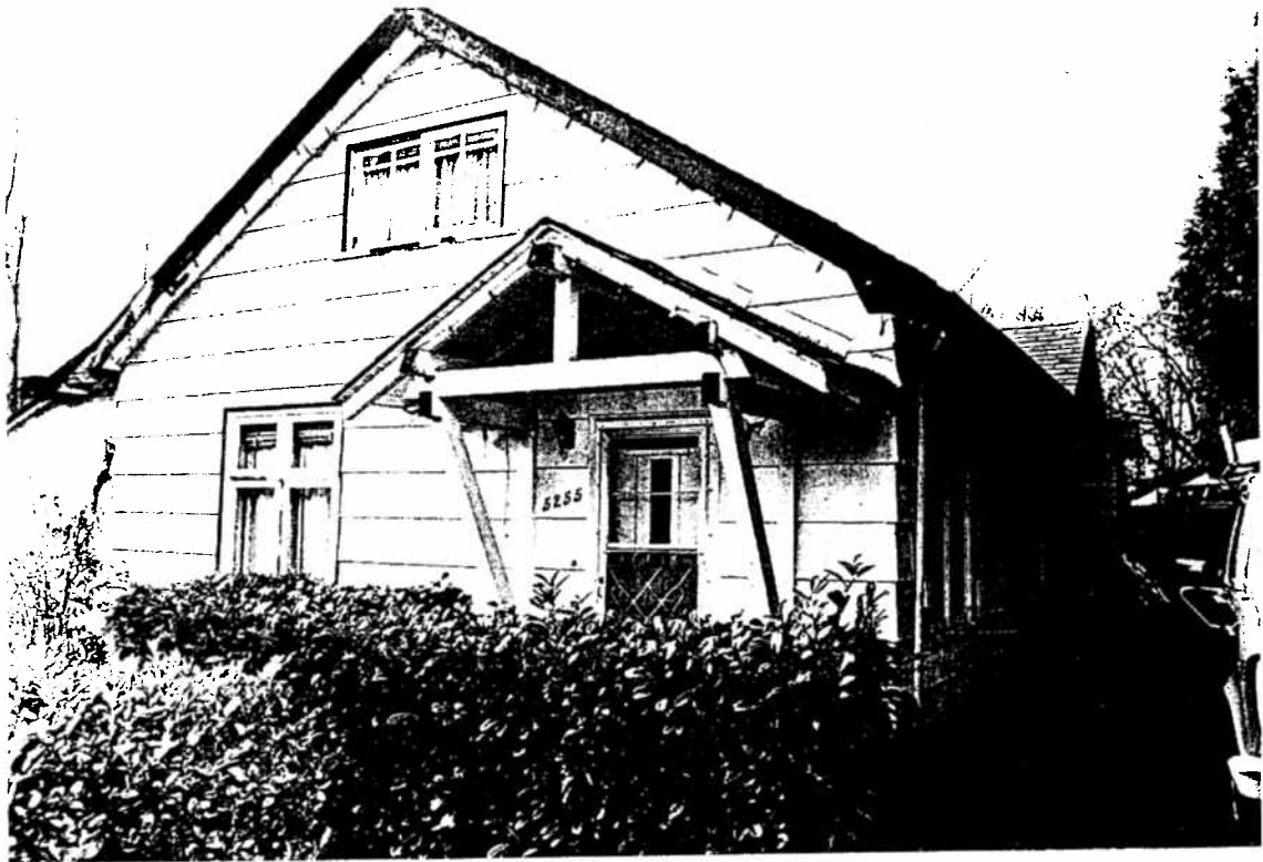
Fig. 3 W.J. Walker House, West facade.
