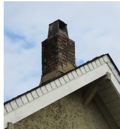
Chimney on west side of the house.
