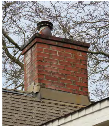
Chimney on east side of the house.
