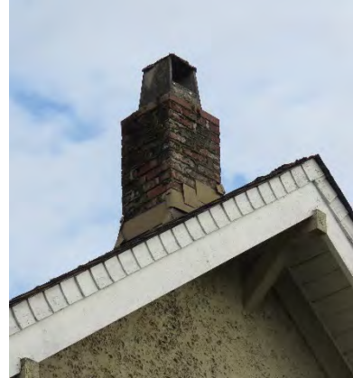
Chimney on west side of the house.
