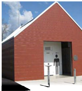
Edmonds Park Washroom
