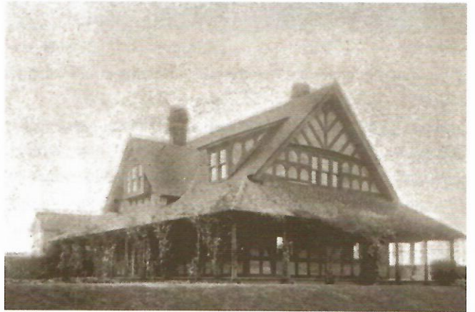
A.J. Dana Residence, Vancouver
