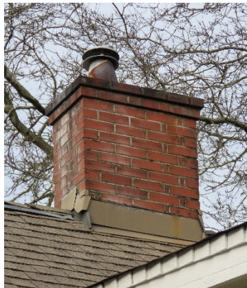
Chimney on east side of the house.
