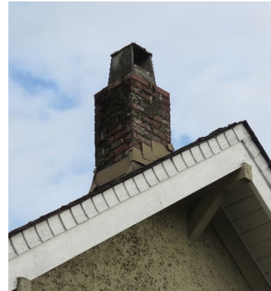
Chimney on west side of the house.
