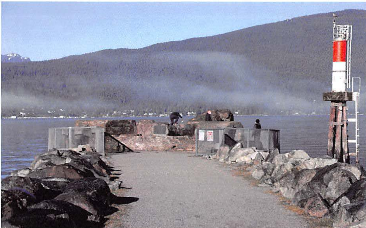
Remains of the sawmill burner from the North Pacific Lumber Mill at Barnet Marine Park
