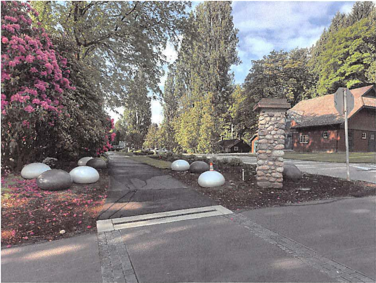
Extant gate post adjacent to the entry driveway to the Burnaby Art Gallery parking lot
