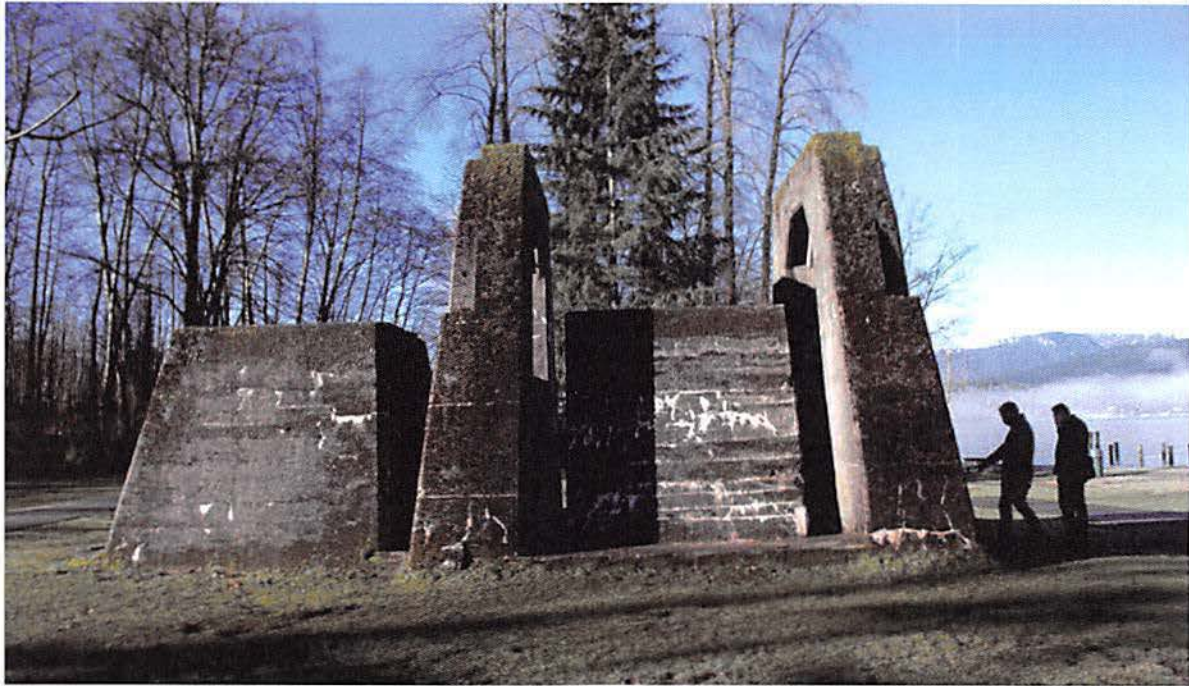
Engine stand base from the North Pacific Lumber Mill at Barnet Marine Park.
