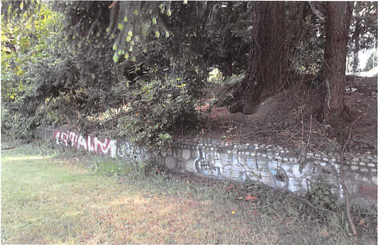
Flanking wall of the Central Park Entrance Gate feature
